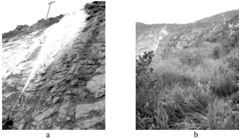
Fig.4. Supporting of bench elements in ultimate position by applying the polymer cover (a), by creating the sod layer on safety berms (b)
